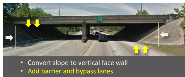
Fig. 11 – Modification of existing bridge end span slopes for PFDI conversion
